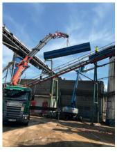
Photo: The new feedstock conveyor was produced at Forestia this summer, being installed during summer maintenance.
